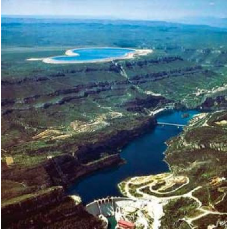
The 635-MW La Muela pumped-storage plant in Spain is being expanded with the addition of a second powerhouse, 852-MW La Muela 2. Iberdrola anticipates that this plant will begin operating in 2012 to help firm the variability of the utility's extensive wind capacity.
